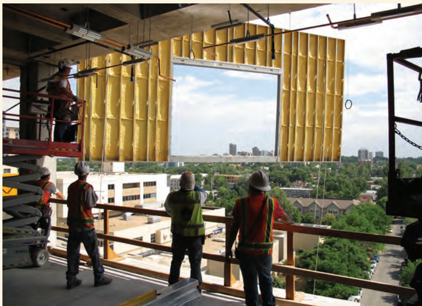
Installation of a prefabricated exterior wall panel.
